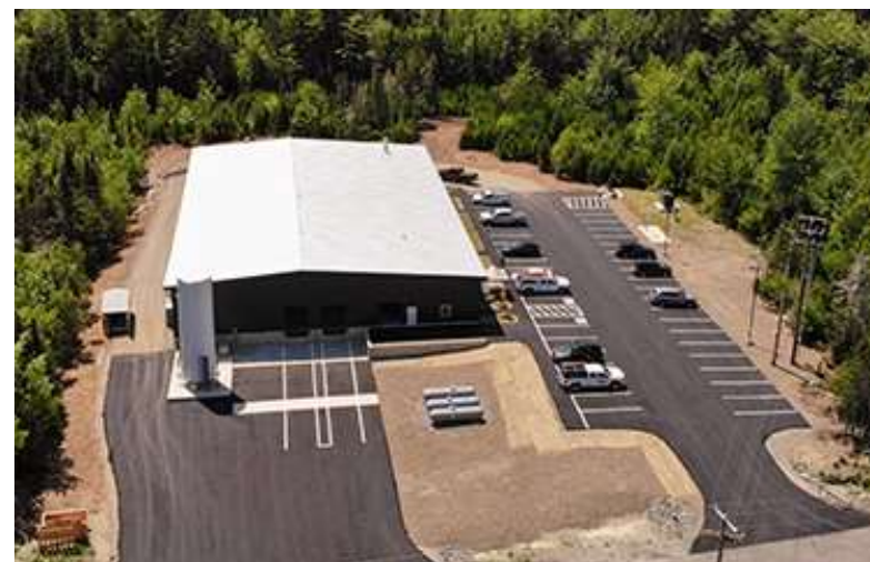
An Example of a small-scale value-add food manufacturing facility (Greenhead Lobster in Bucksport, ME). Photo Source: Greenhead Lobster
